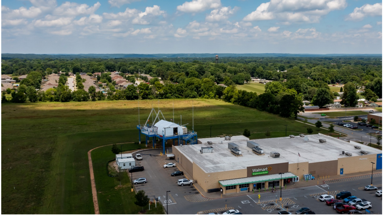
Figure 21 - Walmart store in Arkansas with Zipline cargo port attached.
